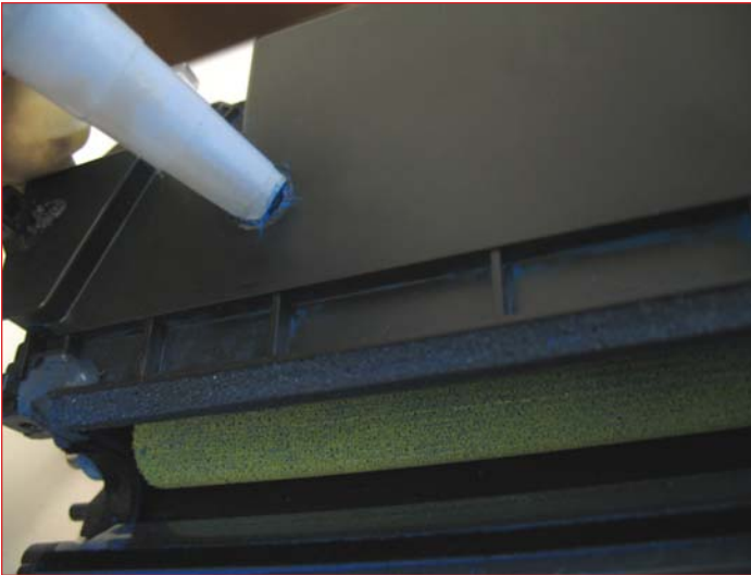
71. Refill the cartridge and cover the opening with sealing tape or a Fill Plug Seal Adhesive .
